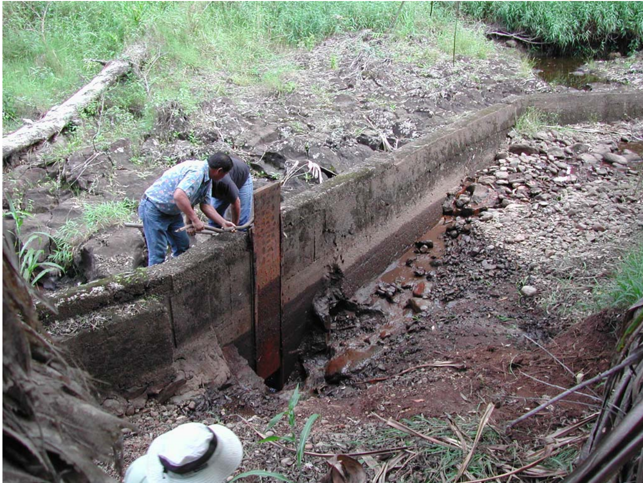
Sluice gate opening is 17-in(W) x 14-in(H)
