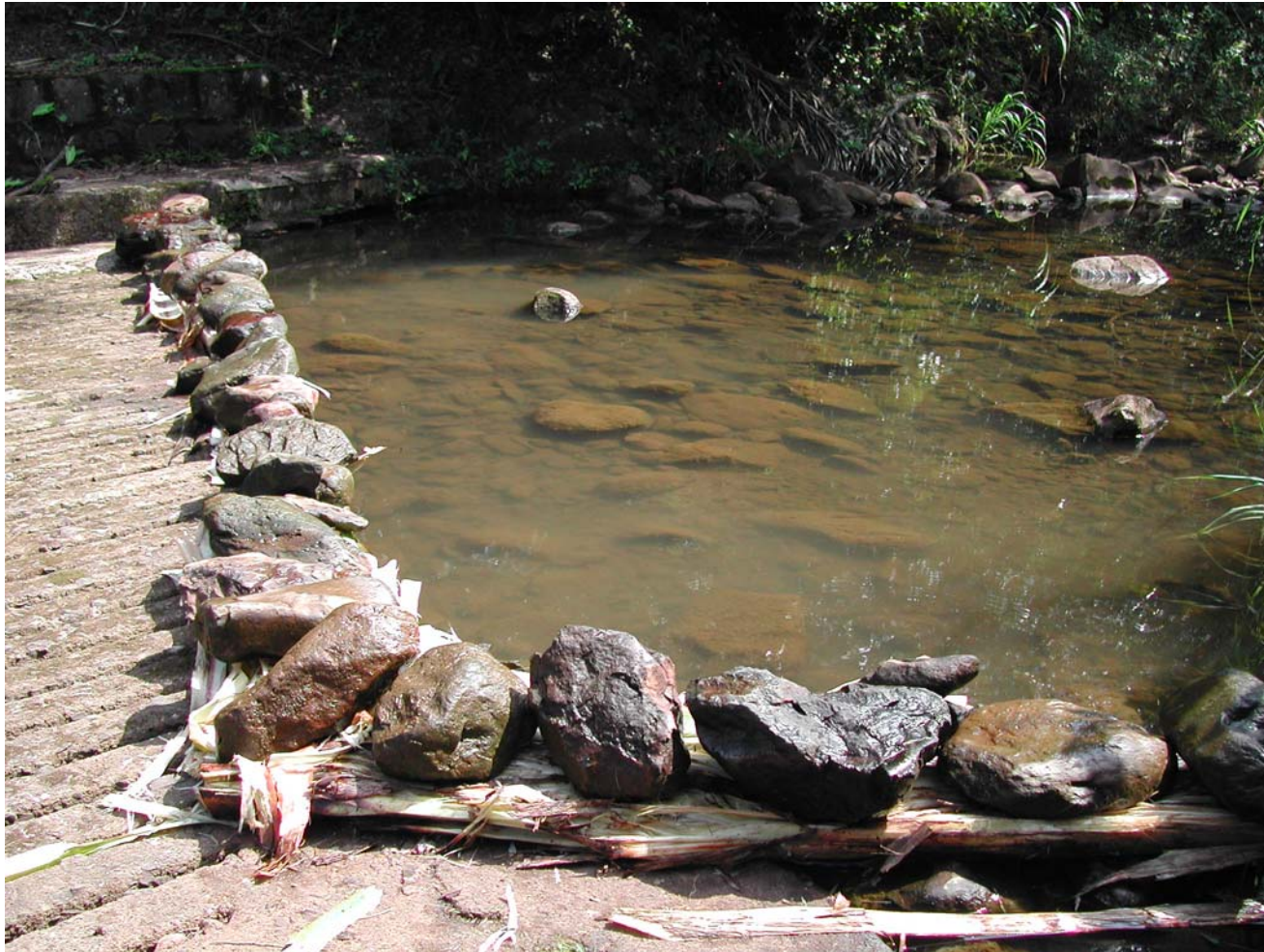
Berm consists of boulders stacked on top of banana stumps
