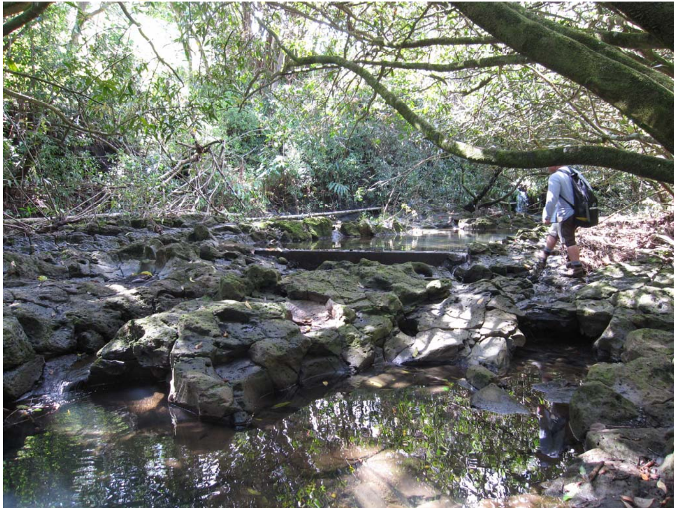
Diversion dam where Waiokamilo and Kualani streams converge
