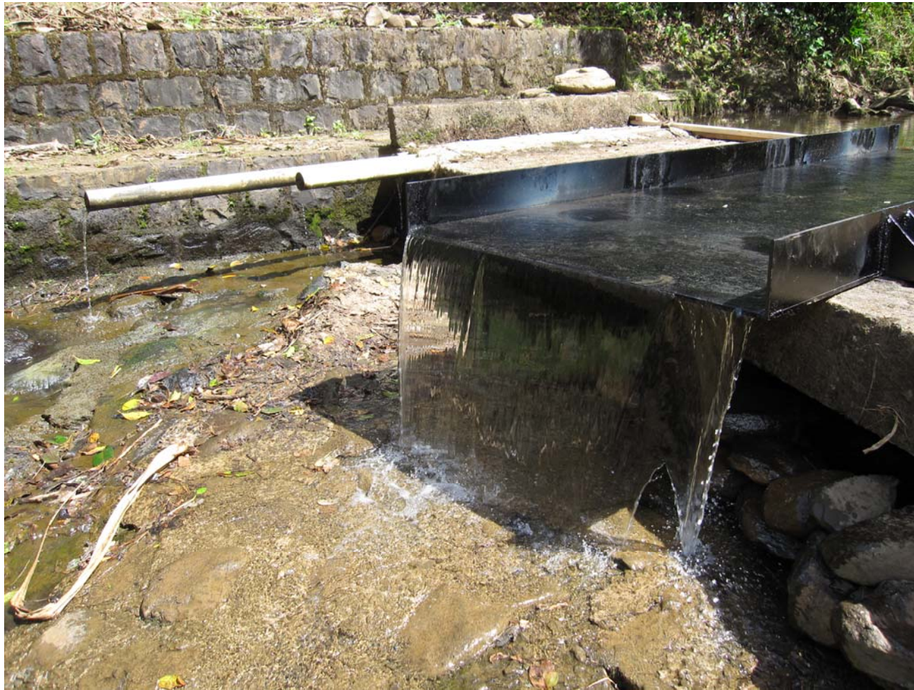
First water flowing past the low flow bypass channel
