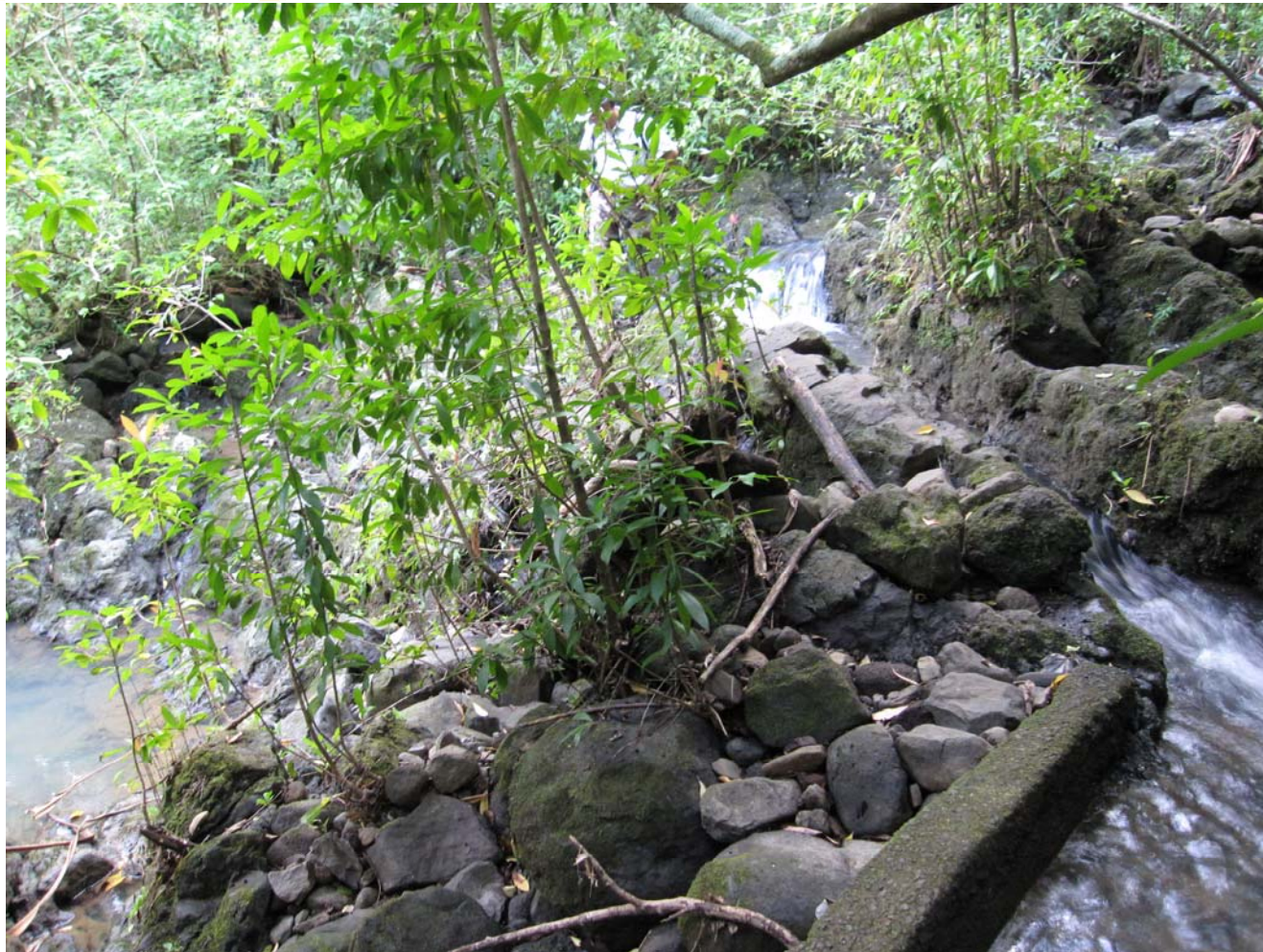
Diversion on Piinaau Stream for the arboretum
